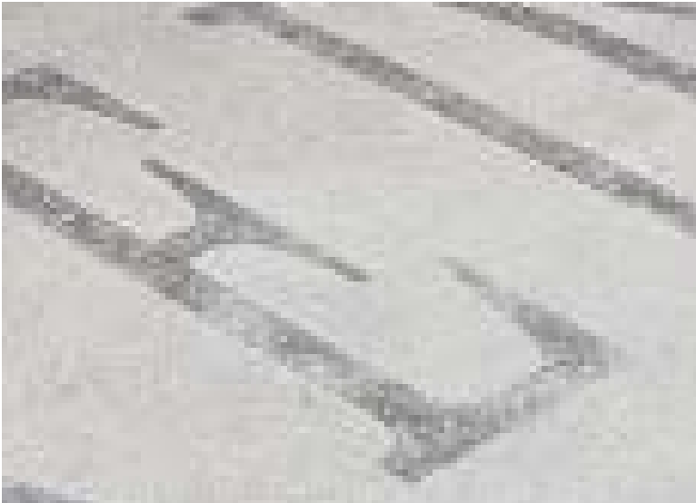
existing concrete with engraved signages
