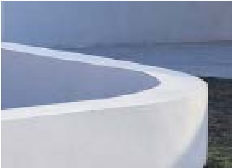
curved concrete wall
